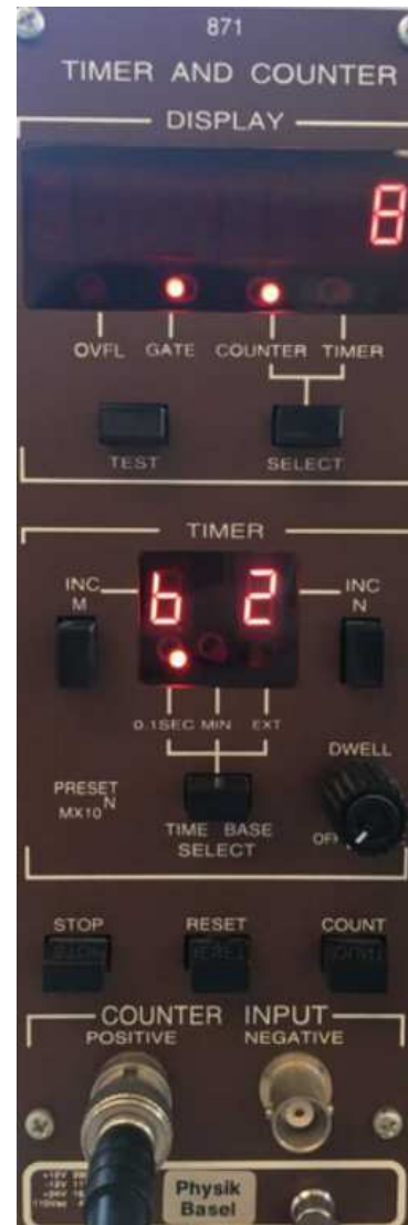
Figure 1.6: The counter is located in the rack with the high-voltage power supply and amplifier. In the center of the counter, a measurement duration can be preset, during which events will be counted.
